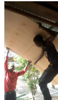
The corridor ceiling under repair
